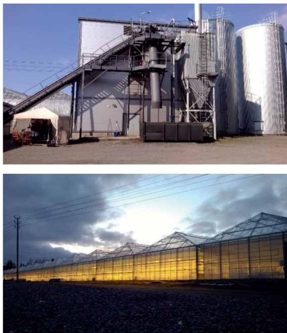
Figure 1. Photographs from the bench scale CO 2 -capture test at the site of a thermal power plant and greenhouse (Photos: Teijo Linnanen)
