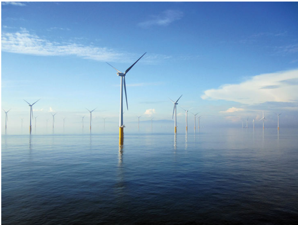
Figure 7 London Array Wind Turbines. Model: SWT 3.6-120, 3,6MW (London Array Ltd., 2013)
