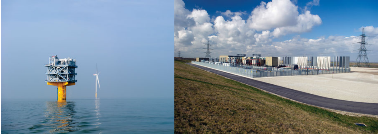
Figure 8 Offshore Substation (London Array, 2013)
