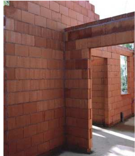
FIGURE 5. Brick masonry construction. (Wienerberger 2014)
