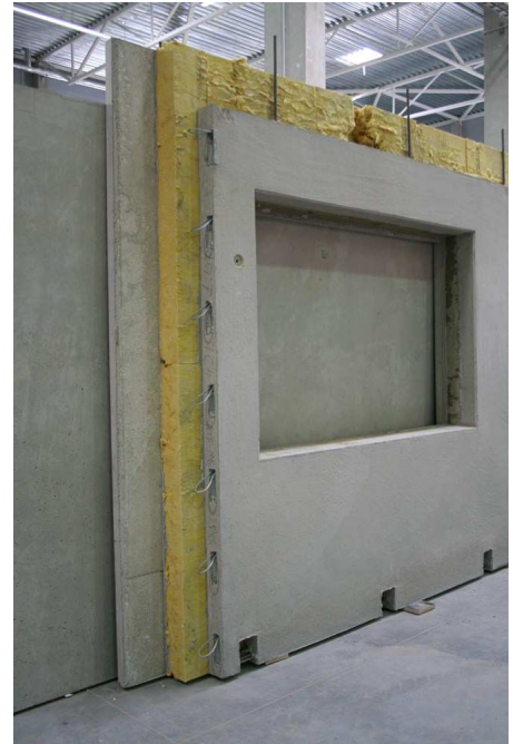
FIGURE 7. Concrete sandwich element (Weckenmann 2014)
