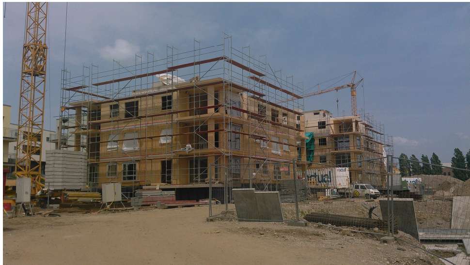
FIGURE 2. CLT construction site in Graz
