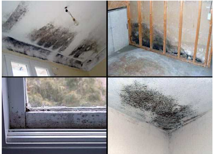
FIGURE 14. Mold growth in thermal bridge areas (Beodom 2014)
