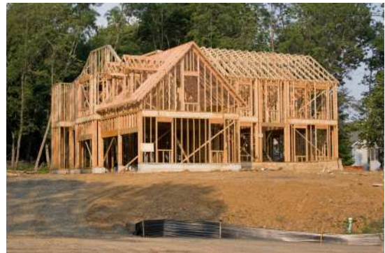
FIGURE 4. Timber frame construction (Buildinganddiy 2014)
