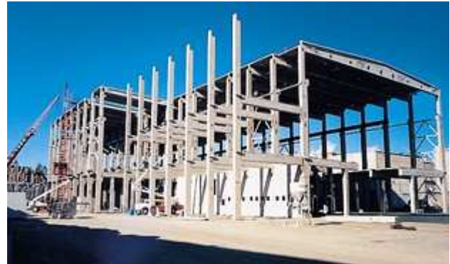
Figure 6. Concrete construction site. (Aaro Kohonen FMC Group, 2014)
