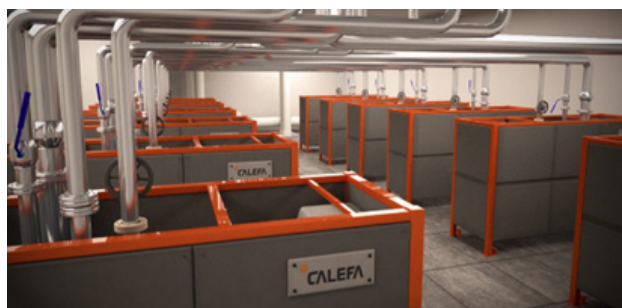
FIGURE 30. Calefa heat pumps at Yandex data centre in Mäntsälä, Finland (Picture courtesy of Calefa Oy)
