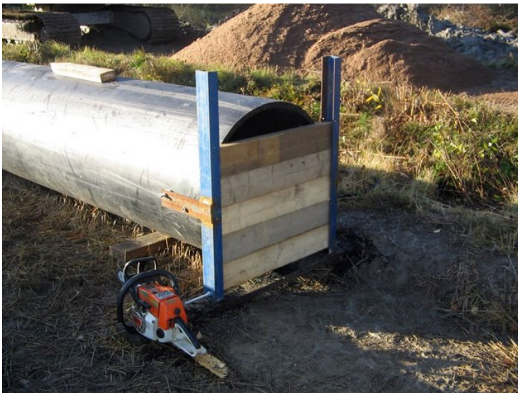
Figure 7. A stop log dam (Hulkianjärvi 2009.).
