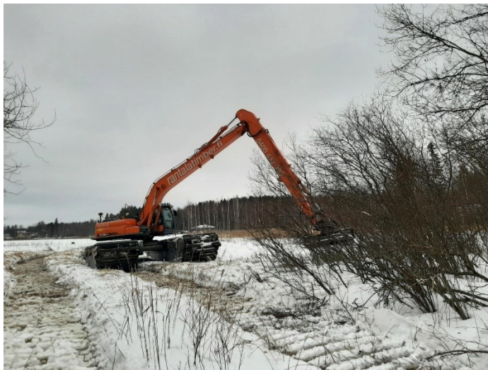
Figure 4. Dredging with a long-boom tracked pontoon machine (Eveliina Sulo, 2024.).
