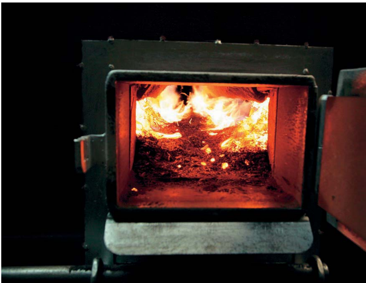
Experimental combustion of the Common Reed in the carburation furnace of Björkboda Manor. The Common Reed burns without problems together with the main fuel which is wood chips, only the amount of the ash generated differentiates it from pure wood fuel. Photo: Sami Lyytinen.
