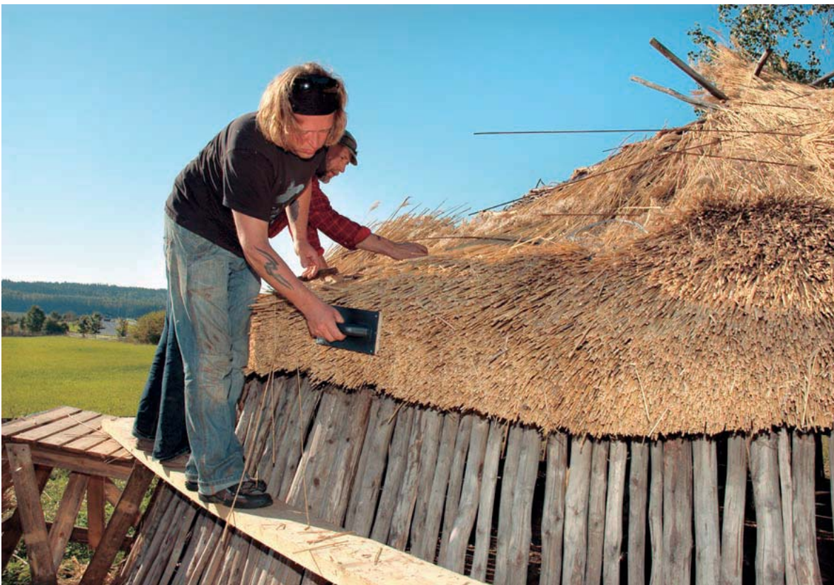
The building of a reed roof was introduced on a course organised by the project "Reed Strategy in Finland and in Estonia" in Turku in the autumn of 2006. Photo: Martti Komulainen.
