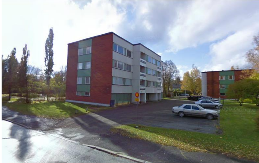
Figure 1 The outlook of the project buildings
