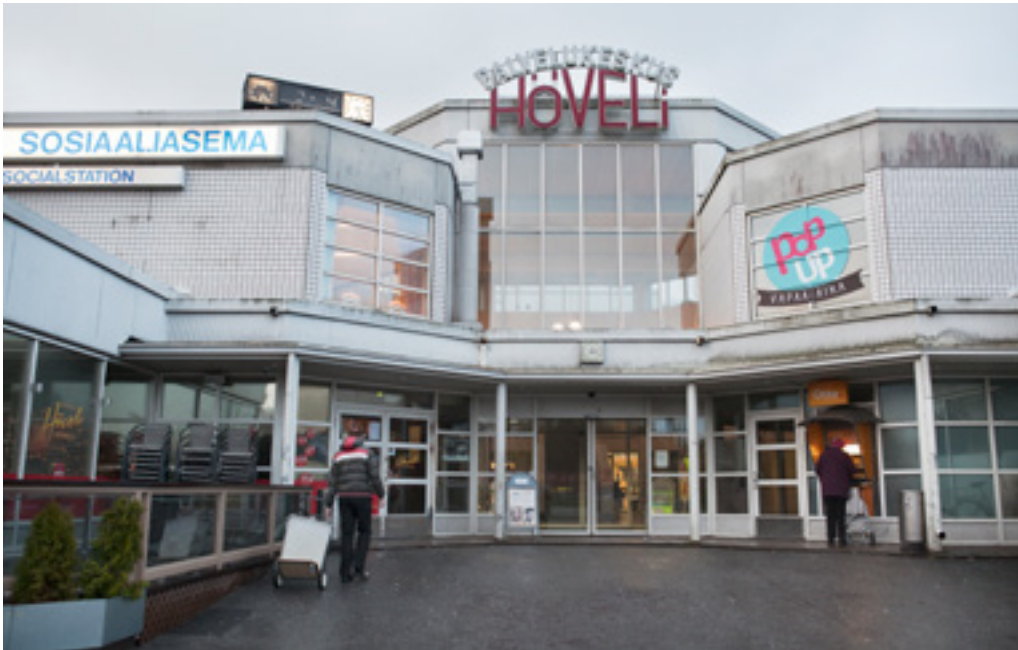
PICTURE 11. Service centre Höveli.
