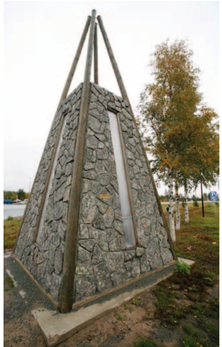
Field stone at monumental art - Polar Circle pyramid -landmark in Rovaniemi, northern Finland. Photos: Urmas Volmer.
