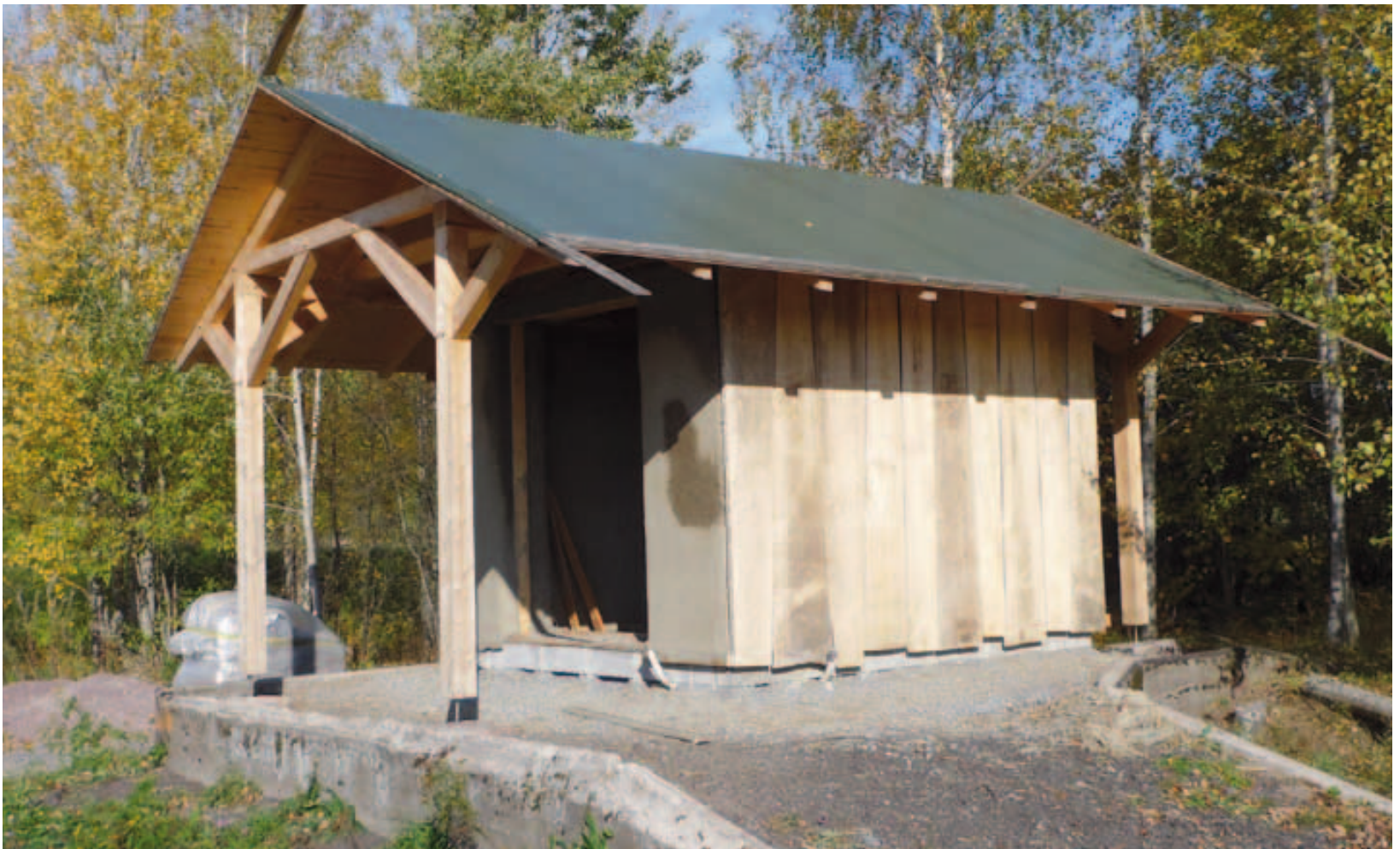
First layer of clay and panels on sides. Photo: Kasper Järnefelt.
