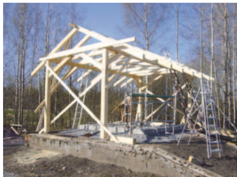
Roof / frame construction. Photo: Kasper Järnefelt.
