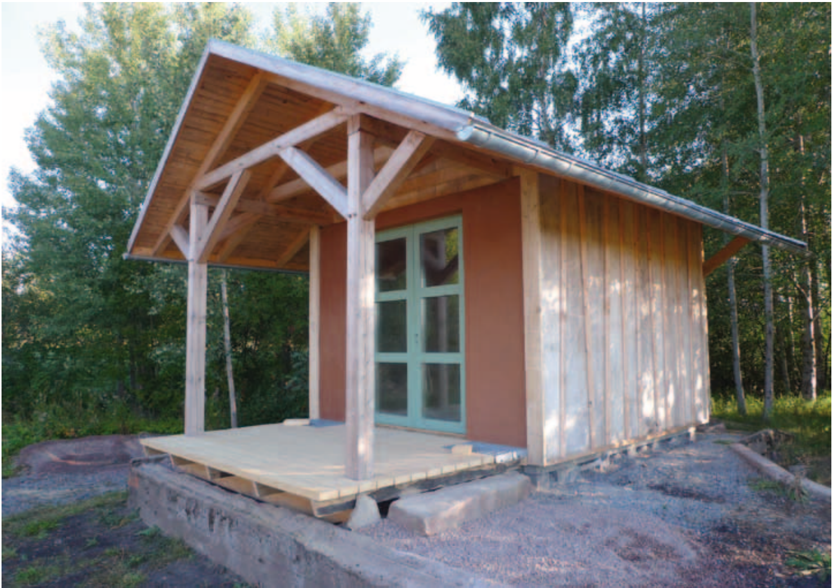
Finished with clay/lime plasters and 100% Rheinzinc metal roof. Photo: Kasper Järnefelt.
