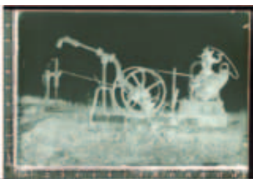
Photo 6: Motorised stone drilling machine. Field technique from the early 20th century (ERM Fk 2133:6642).
