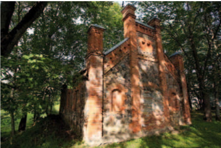
Õisu estate winery from the 19th century - the historicistic building from field stones and bricks.
