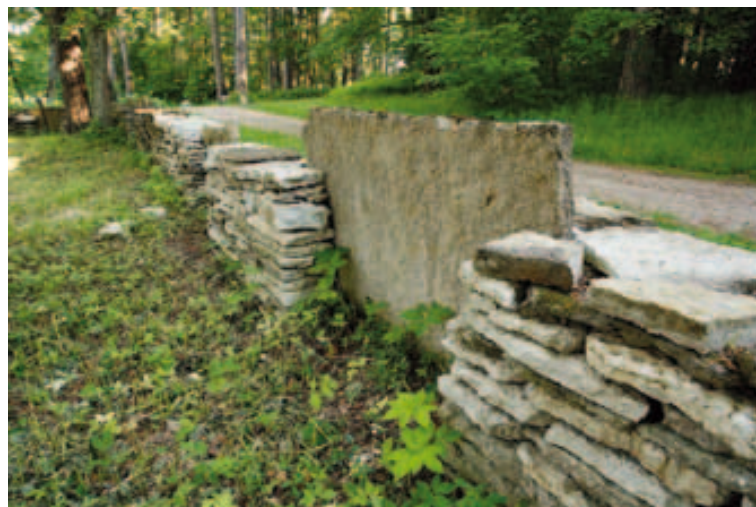
For many future masons, a stone wall has often been the first source of experience. A restored wall built from limestone at the Estonian Open Air Museum. Many walls in northern Estonia were extended with large vertical slabs of limestone.
