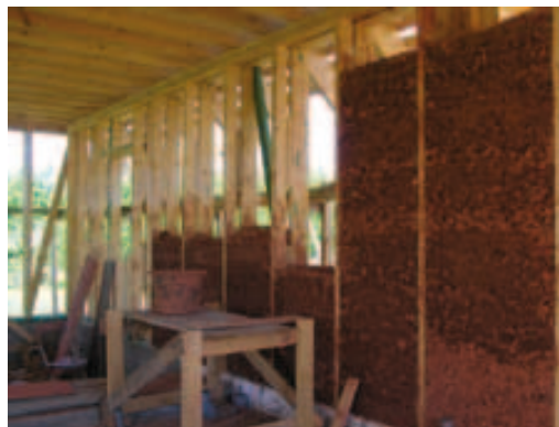
Picture 1: Single-family house in Ihamaru with timber-framed walls in filled with lightweight clay with wood chips built in 2006 Photos: Marko Kikas.
