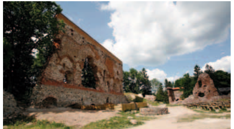
Fieldstones have been used in construction in southern Estonia for a long period of time. The Viljandi castle of Teutonic Order that was mainly erected in the 13th and 14th century was the second largest after Riga in the historic Livonia. Picture from the ruins of the convent house.
