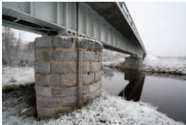
An example of technically demanding fieldstone masonry. A bridge over the River Mustjõgi near Saru in Valga County, on the former Valga-Ape narrow-gauge railway, thought to be built in 1919. Now in use as a road bridge. Photos: Urmas Volmer.
