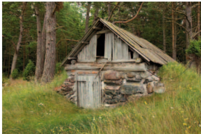
A building constructed of fieldstone will likely end up being extremely long-lived and picturesque even if the builder is DIY and relatively inexperienced. A store cellar on Hiiumaa Island near Kalana port. Photo: Urmas Volmer.
