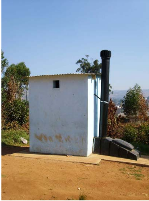
PICTURE 2. South African dry toilet model Enviroloo at the Msunduzu Sports Grounds. Picture: Sini Haimi
