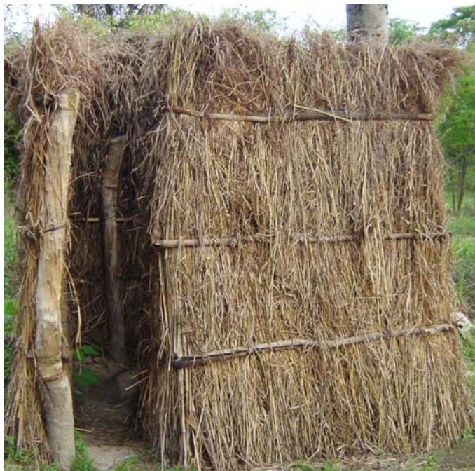
PICTURE 2. Pit latrine with temporary grass structure. Picture: Sari Huuhtanen
