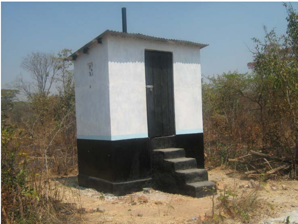
PICTURE 2. Model of standard dry toilets built in Kaloko. Picture: Emmanuel Mutamba
