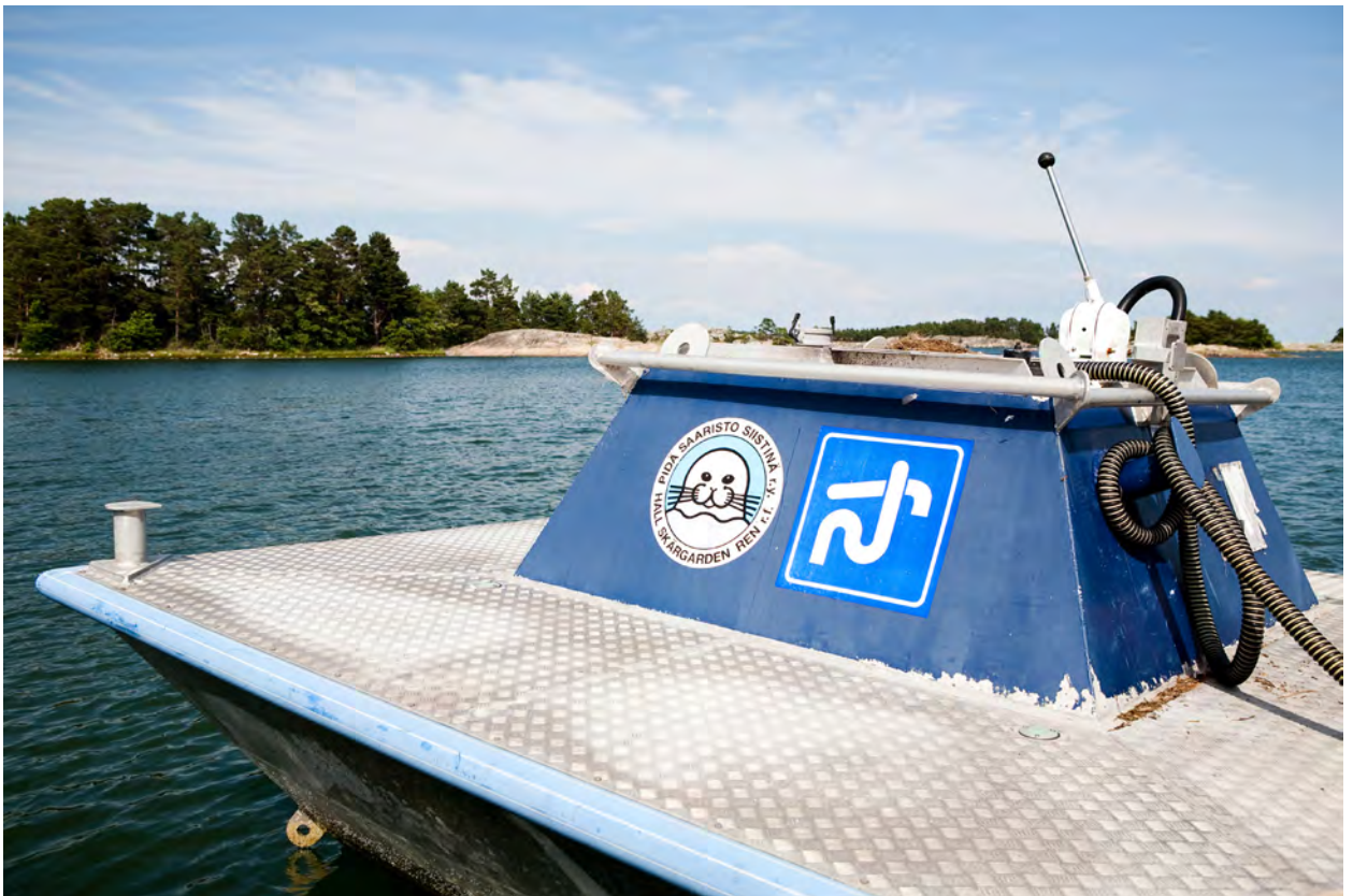
A floating septic tank pump-out station. (Photo: Keep the Archipelago Tidy Association)
