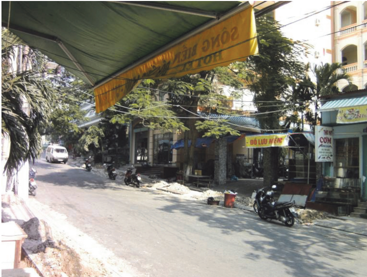
PICTURE 4. In Cat Ba town lots of investments has been made for new hotels. Our research revealed that the infrastructure in the town is poor and not ready for the sudden increase of tourists. (Photo: Jari Hietaranta)
