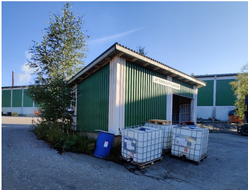
Figure 10. Waste collection station located in the sawmill yard.
