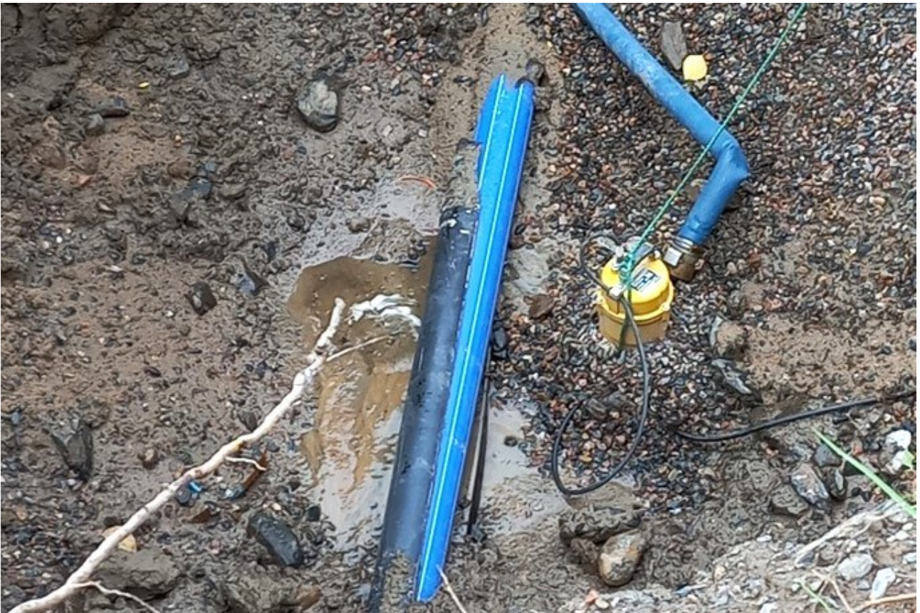
IMAGE 4. A new pipe and the old split pipe in the pit [5].
