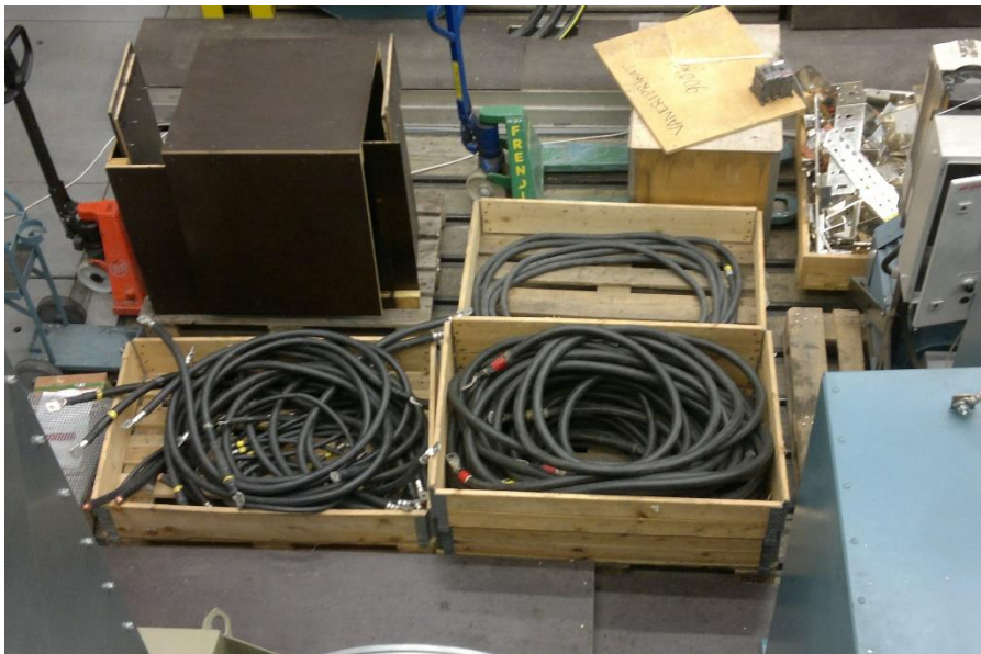
Picture 2. Cables in the middle of motors, ground plan number: 4
