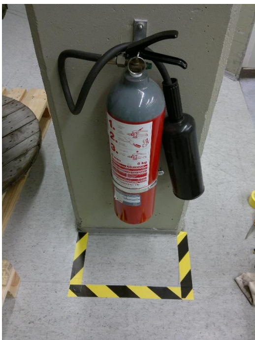
Picture 26. Marking for a fire extinguisher
