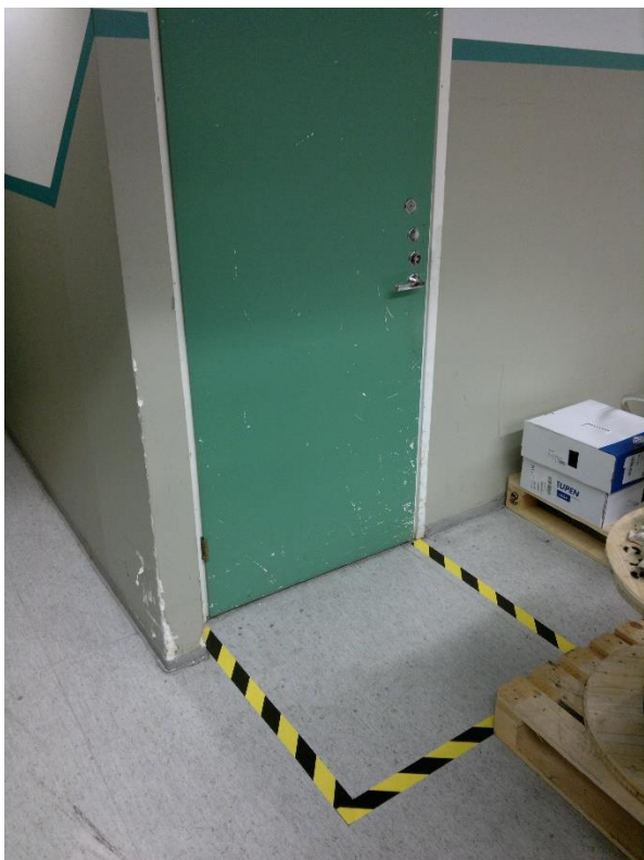
Picture 25. Marking for a door
