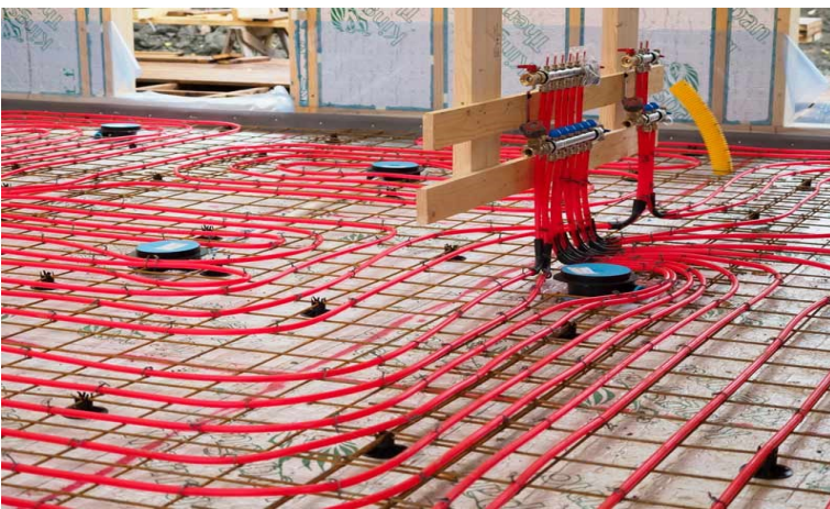
Figure 6: Floor water heating system.
