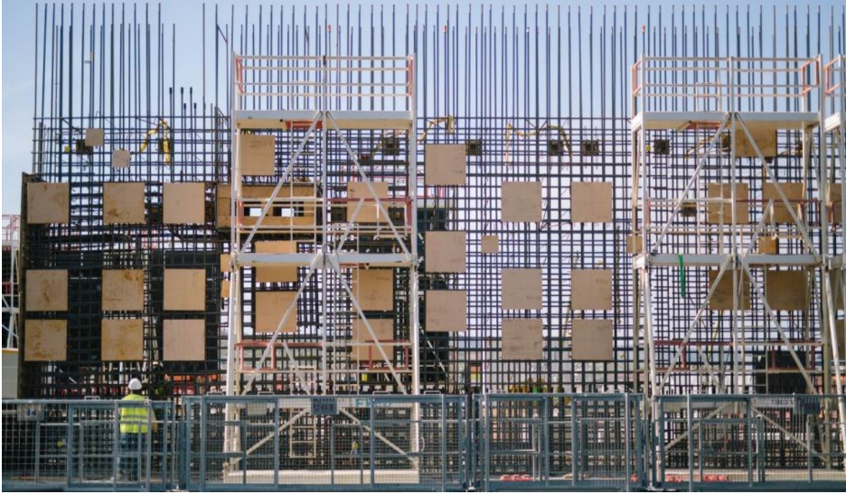
Figure 11. Supporting fixtures are welded into the exposed plates. (iter, 2021)
