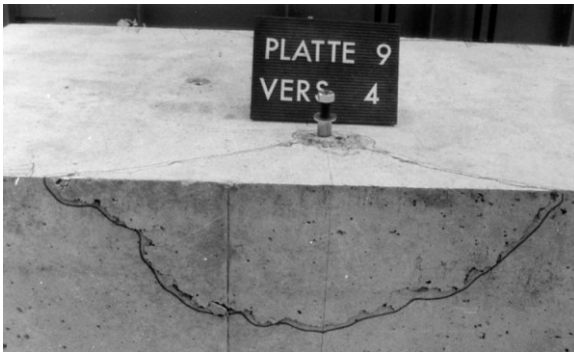
Figure 17. Concrete edge failure. (Eligehausen et al., 2006, p. 112)
