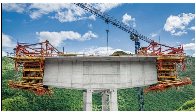
Image 9. Balanced concreting technology (PERI)
