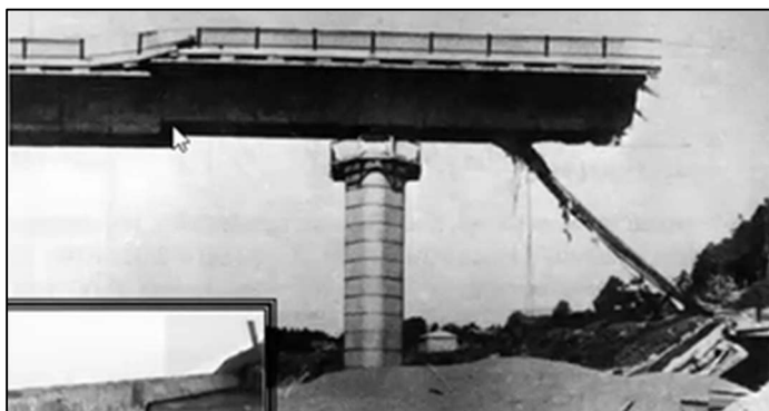
Image 19. The collapse of the bridge over Suhona river (Syrkov 2021)
