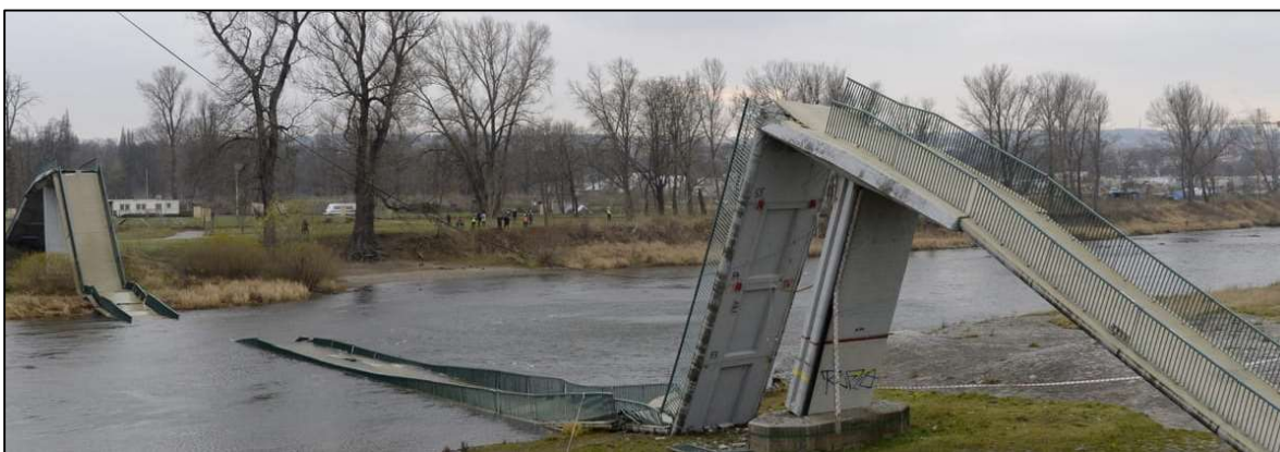
Image 18. The Troja footbridge after collapse
