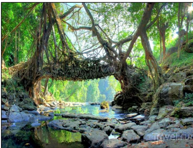
Image 1. “live” suspension bridge in India (Image: Rohit Mordani)
