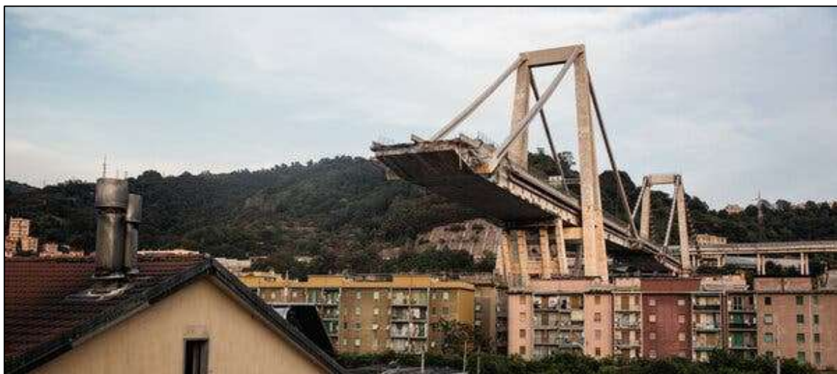
Image 14. Collapsed Morandi Bridge (Image: Nadia Shira Cohen)
