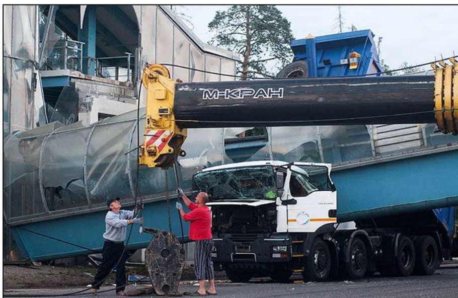
Image 10. Pedestrian bridge collapse on the road M-10 (Interfax 2016)
