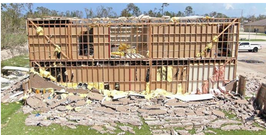
Figure 4. Consequences of wind loads (KORZHIK.NET 2016)
