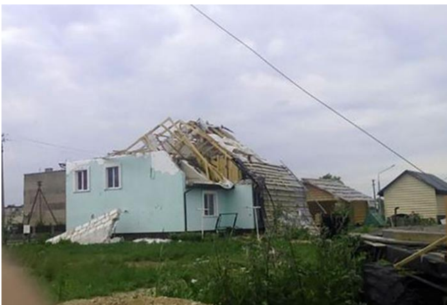
Figure 3. Consequences of wind loads (KORZHIK.NET 2016)
