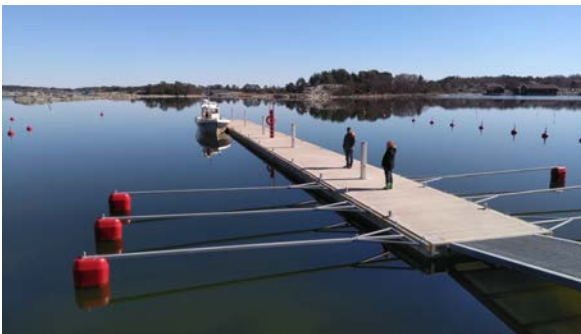
The new jetty at Stenskär
