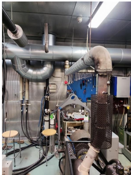
Figure 39. Extractor pipe and laboratory exhaust gas system with the common channel pipe and exit pipe in the background (Author's own).
