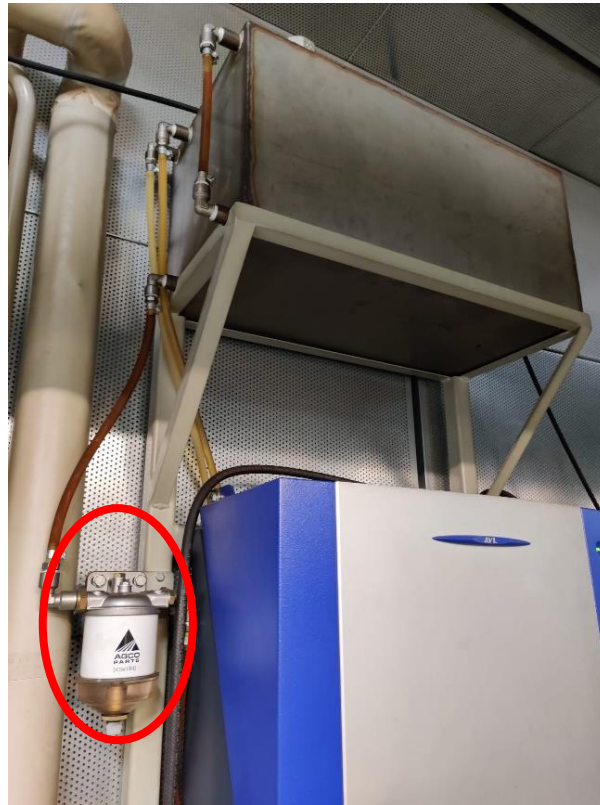
Figure 19. Pre-filter used on the SISU engine – annotated with a red circle (Author's own).
