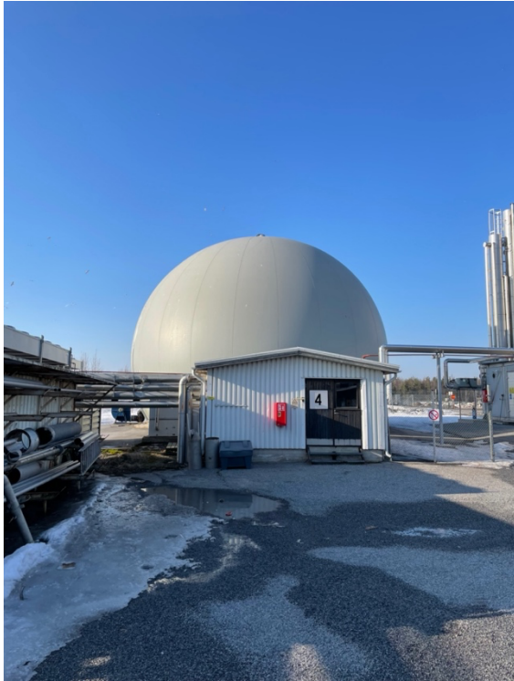
Figure 10. Gas storage at Stormossen Oy.
