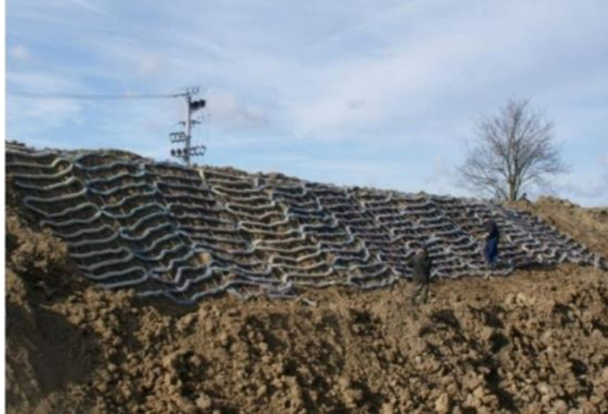
PICTURE 1. Anti-erosion geotextile ropes slope, 09.02.2016. (Nguyen et al., 2021)
