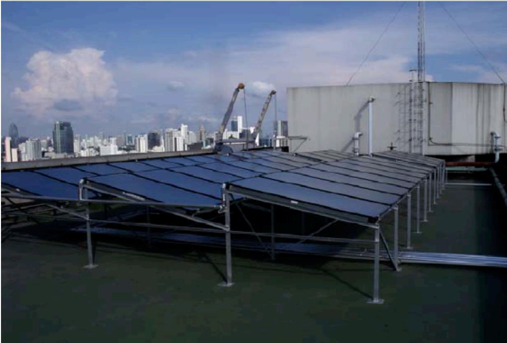
Figure 11: Flat Plate Solar Collectors on the roof top of Royal Orchid Sheraton Hotel
