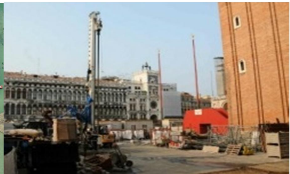
Image 14: Reparation of San Marco square
