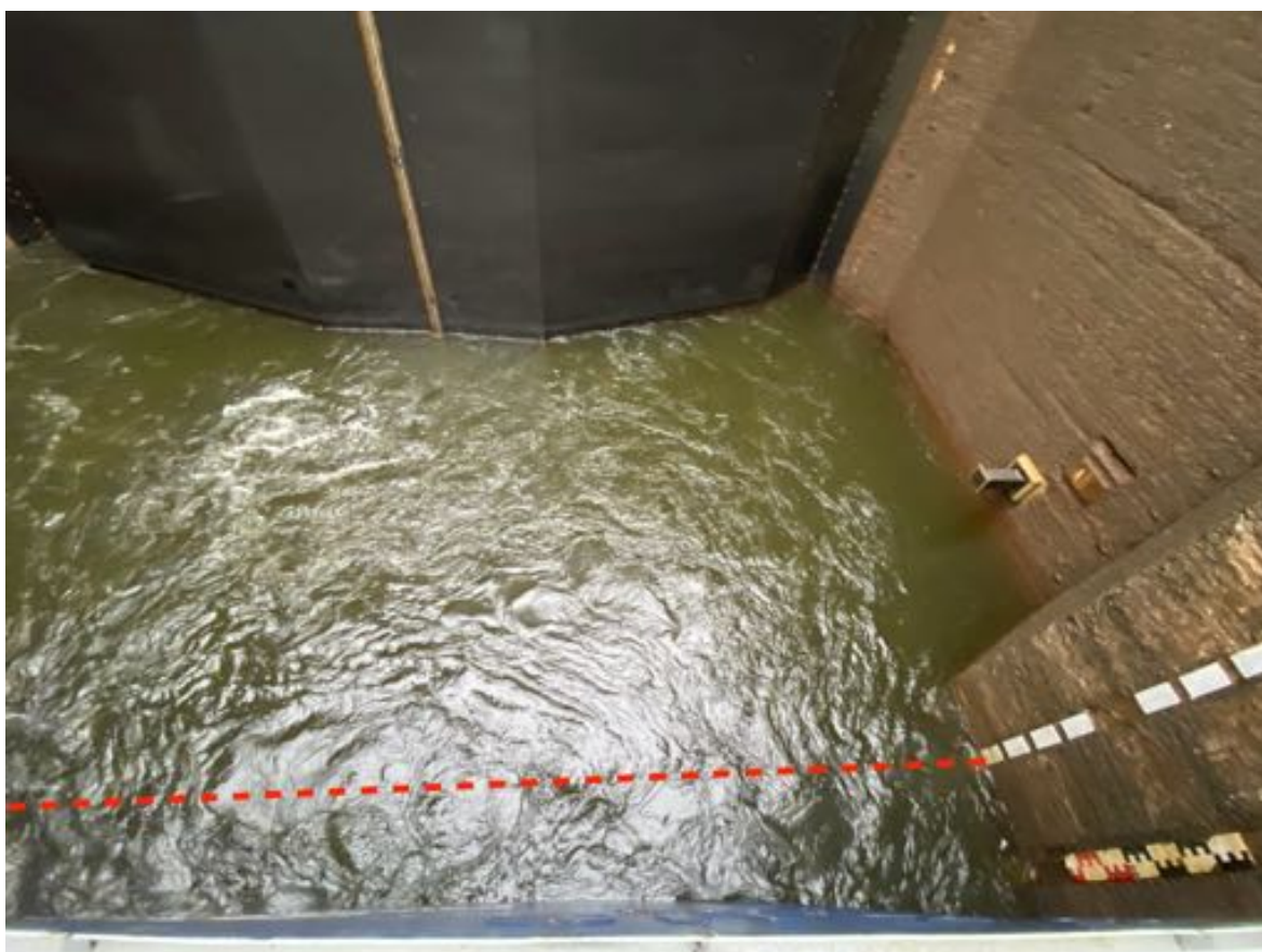
Figure 12: Limits of a vessel in a lock for a saimax vessel. MV Nina inbound at low-water. (Antti Tasala, 2021)
