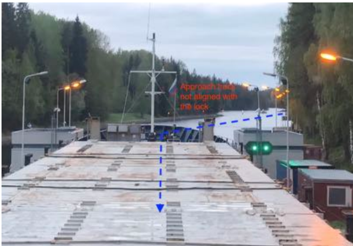
Figure 38: Note Cvetotchnoe lock entrance angle in outbound traffic. MV Nina inbound in the picture. (Antti Tasala, 2021)
