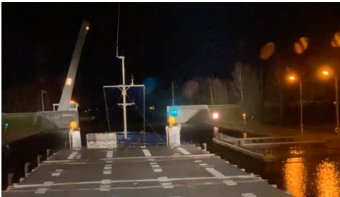
Figure 24: Kansola northern pier on starboard side for temporary mooring. Similar pier at southern side after bridge. Visible on port side forward quarter. (Antti Tasala, 2021)
