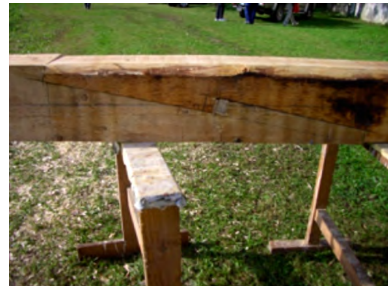
Figure 3.30. The finished joint.
