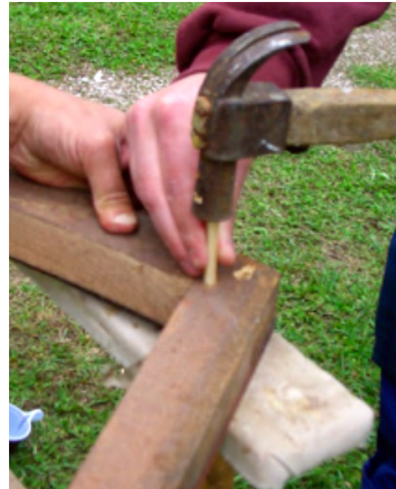
Figure 3.34. A new peg is being pounded gently into the casement of a window.
