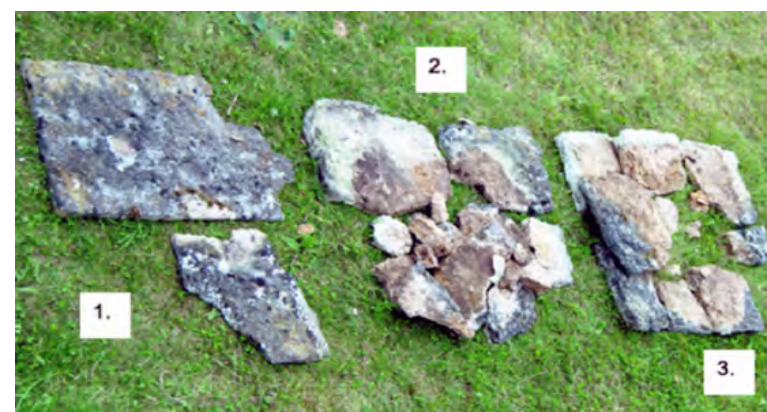
Figure 2.14. Dismantled stones from gatepost: top level (1), second layer (2)—middle part, and right—third layer from top, bottom part of gatepost profile (3).
