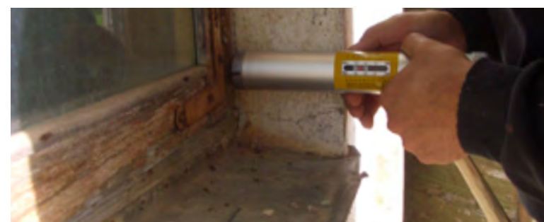
Figures 3.15–16. The Pilodyn was tested on timber with various degrees of decay.
