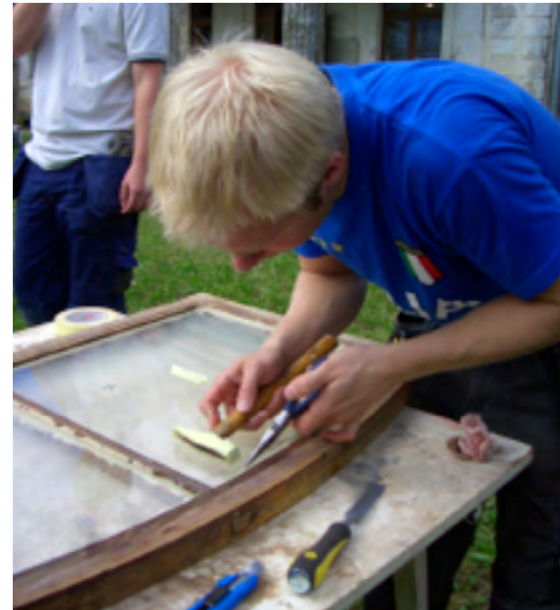
Figure 3.36. Nails are being inserted. The small hammer is wrapped in masking tape to avoid scratches on the glass.
