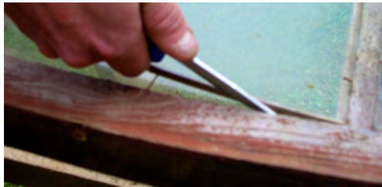
Figure 3.33. A glazing bead is being removed.
