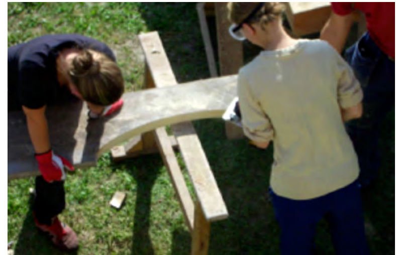
Figure 3.42. Consoles for the upper hall cornice are being made.
