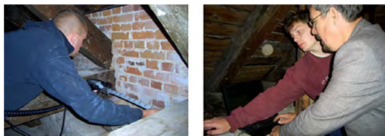
Figures 3.14. One student is drilling into a roof truss while the other is learning to interpret the transmitted information on the computer. Prof. Kalle Pilt, lecturer at Estonian University of life Sciences, (far right) is explaining the curves on his computer screen.
