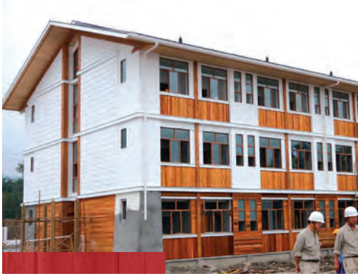
FIGURE 17. XIANG'E PRIMARY SCHOOL IN DUJIANGYAN, 2009
