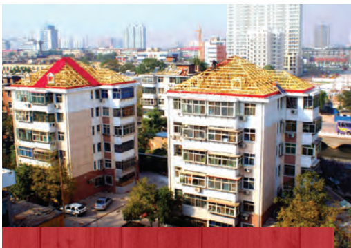
FIGURE 19. WOOD TRUSS ROOFING SYSTEM, SHIJIAZHUANG
