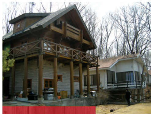
PIc. 1.9 VERY LITTLE DAMAGE ON THE BUILDING AS A WHOLE
