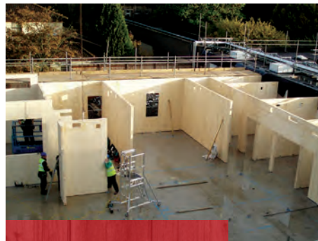
FIGURE 40. NEW STRUCTURAL SYSTEM BY CROSS LAMINATED TIMBER
