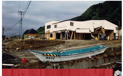
Pic. 1.3 RESTAURANT "HATOU" LOCATED BEHIND
