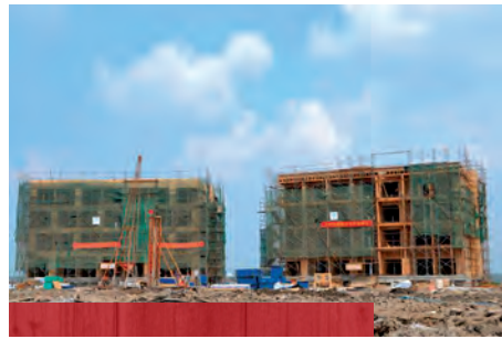
FIGURE 38. LIGHT WOOD FRAME HOTEL SITE WITH 4 STORIES, TIANJIN
