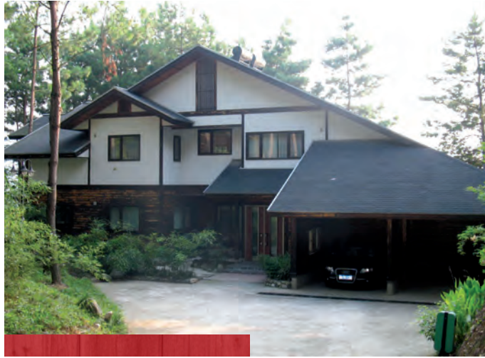
FIGURE 16. WOODEN HOUSE INTRODUCED FROM JAPAN IN 2005, ANHUI
