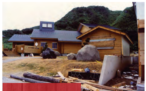
Pic. 1.5 BROKEN CONCRETE WALL
