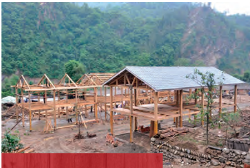
FIGURE 39. THE POST AND BEAM REBUILT HOUSES SITES, QINGCHUAN
