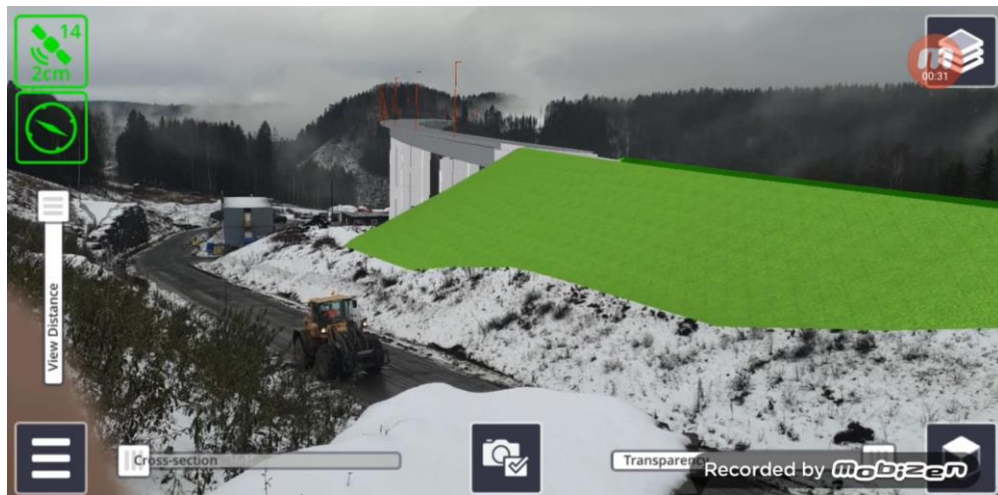
Figure 41: Augmented reality for the bridge location illustrated in its correct coordinates at the site (Copyrights for Sweco company with the permission of the author's use only).
