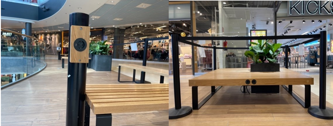
Figure 4. Power sockets in public seats in Koskikeskus. (Lin, 2021)
