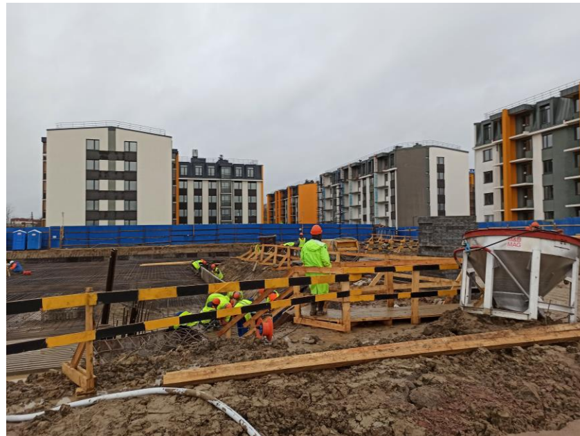
Figure 3.4 Reusable wooden safety barriers around a foundation pit
