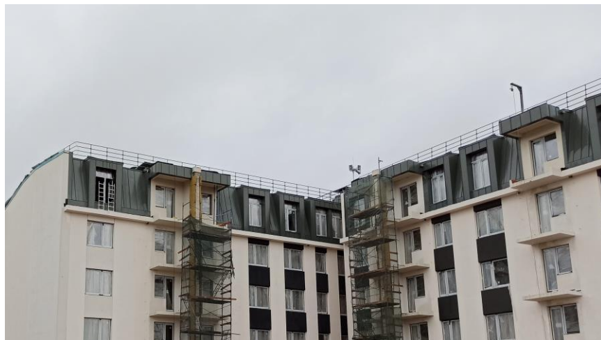
Figure 3.6 Galvanized steel plates roofing
