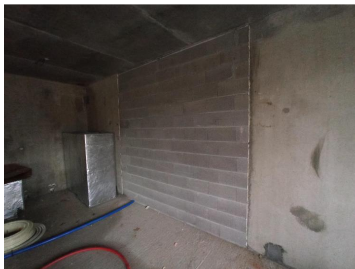
Figure 3.5 Demolishable wall design solution for apartment conjunction
