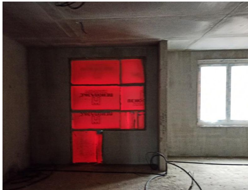
Figure 3.7 Openings covering for temperature control.
