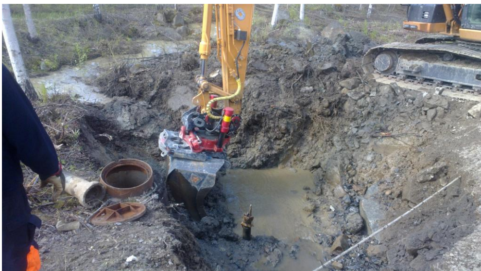
PICTURE 3.1. Excavation happening to find out the leaking point (Chowdhury 2012)
