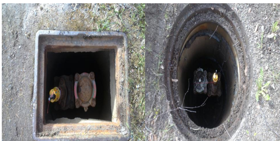
PICTURE 5.1. Noise logger installation inside the fire hydrant (Chowdhury 2012)
