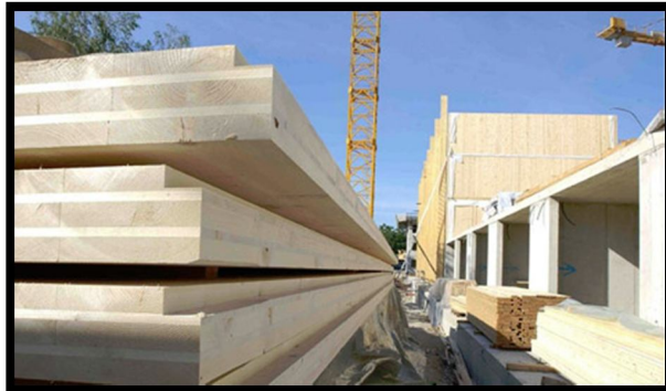
Figure 2.2 Typical CLT products (eni.info internet site, http://www.esi.info/detail.cfm , Natural Resources Canada, http://www.nrcan.gc.ca/science/story/6000 )
