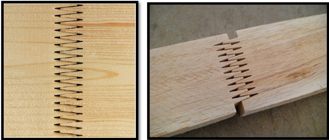
Figure 2.4 Connection with finger jointing (Made-in-China.com, http://www.made-in-china.com/showroom/woodwintimber/product-detailZoKJWfkbrLVv/China-Finger-Joint-Wood.html )
