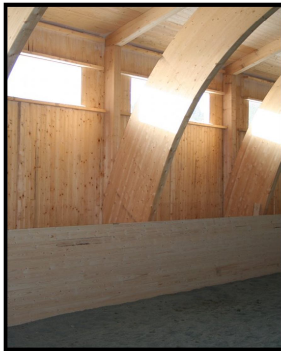
Figure 2.20 Views of the inside structures (Norsk salsenter, http://www.norsksalsenter.no/salsenteret )
