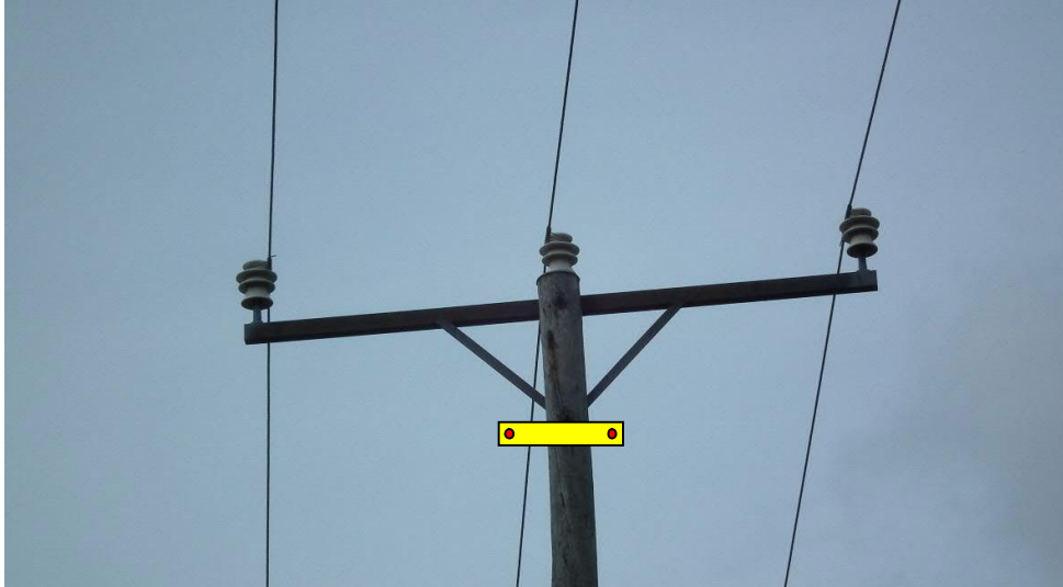
Fig. 1. A typical 20-kV transmission line with three current-conducting wires
