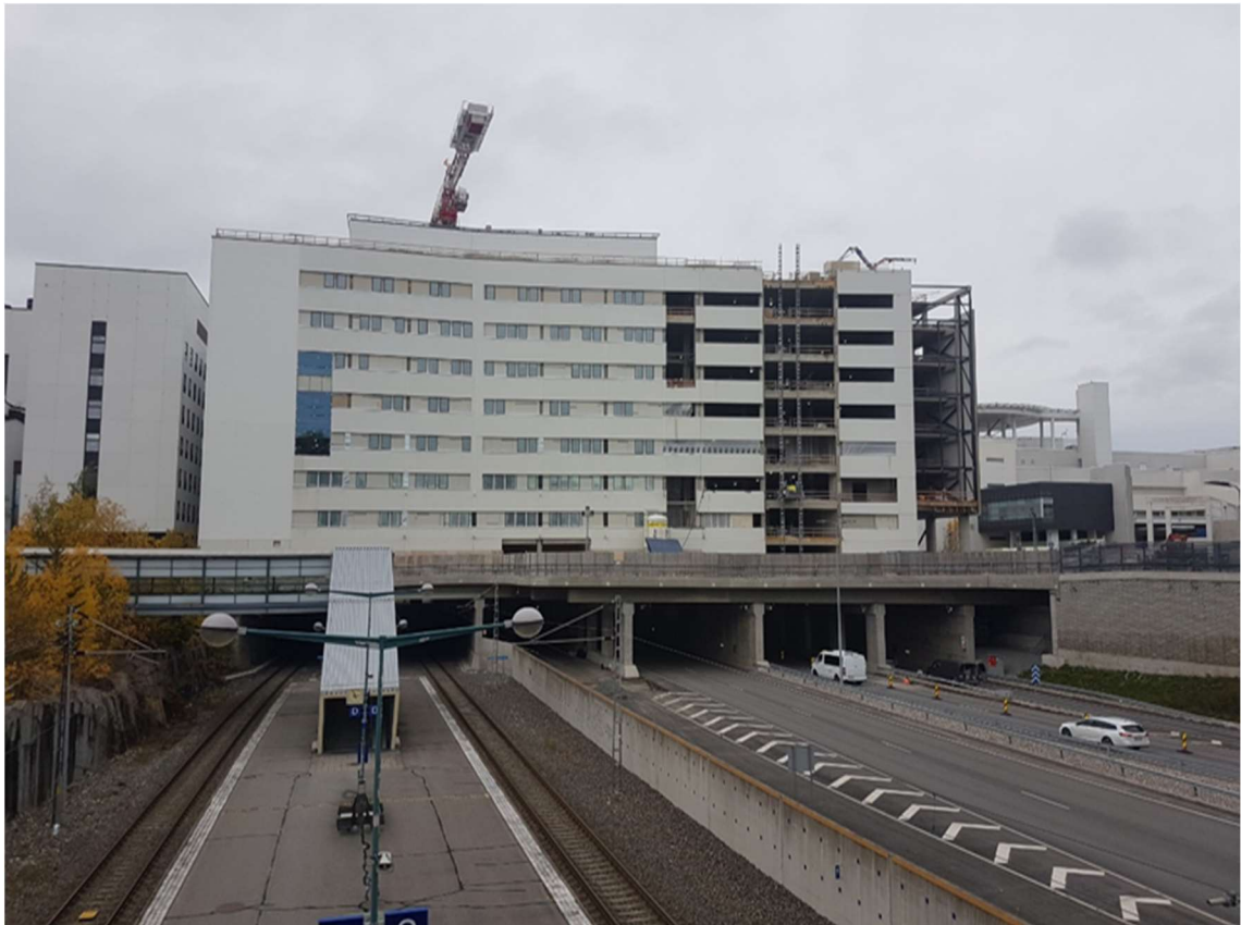
Picture 1. T3-project shot from the direction of Tykistökatu 15.10.2019.
