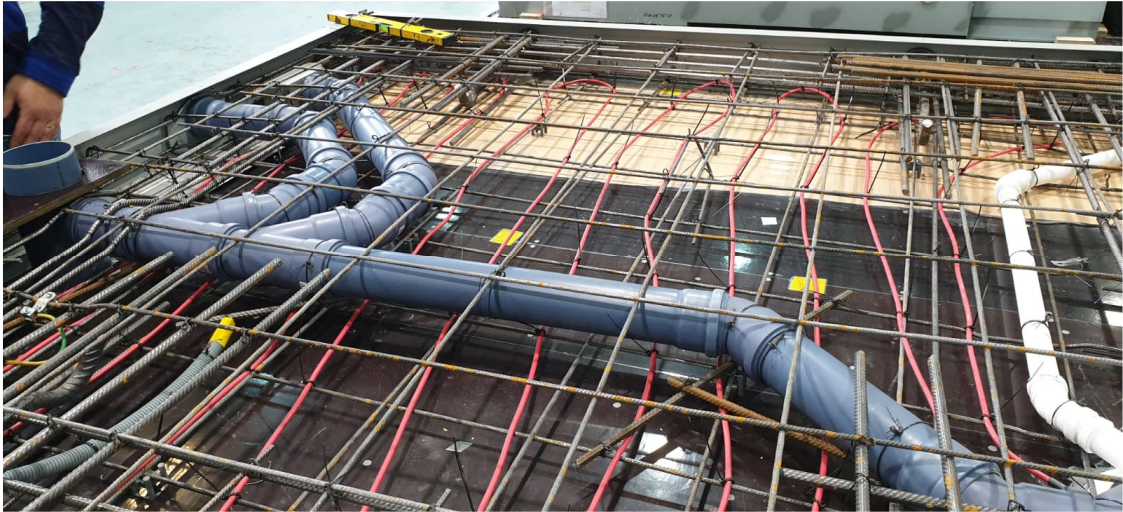
Figure 15: Drainage pipes and electrical heating cables installed into the slab cast.
