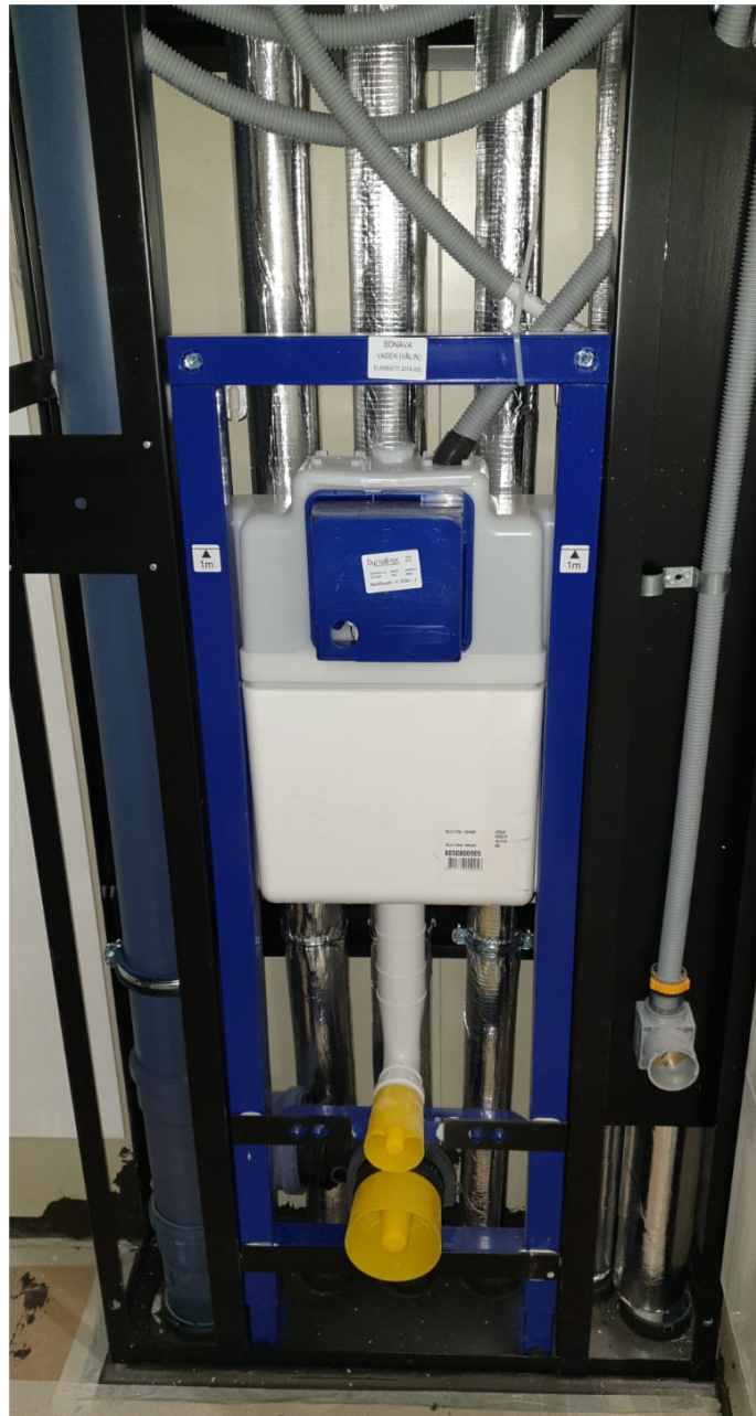
Figure 6: Left-handed pipe shaft installation.
