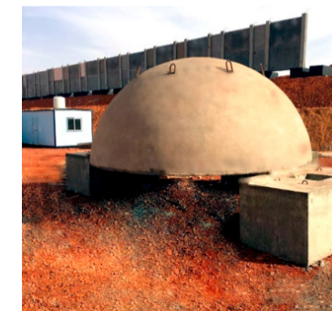
Figure 2.4 precast dome for cathedral (By the Author)
