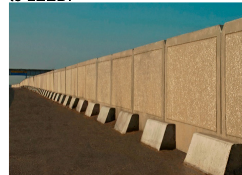
Figure 2.3 Example of precast movable fence (By the Author)
