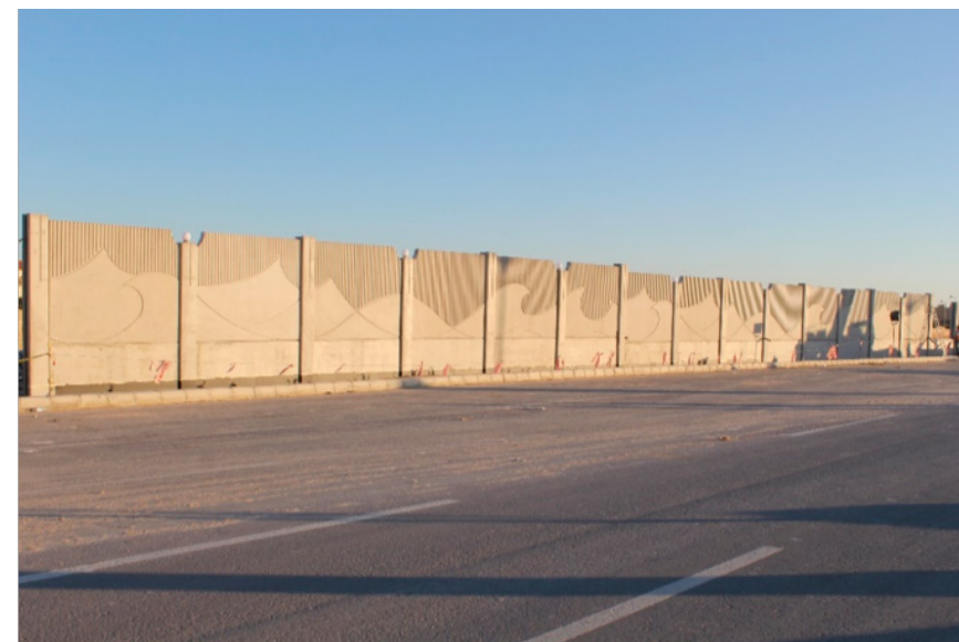
Figure 2.6 Precast Fence for a construction site in New Alamein City (by the Author)
