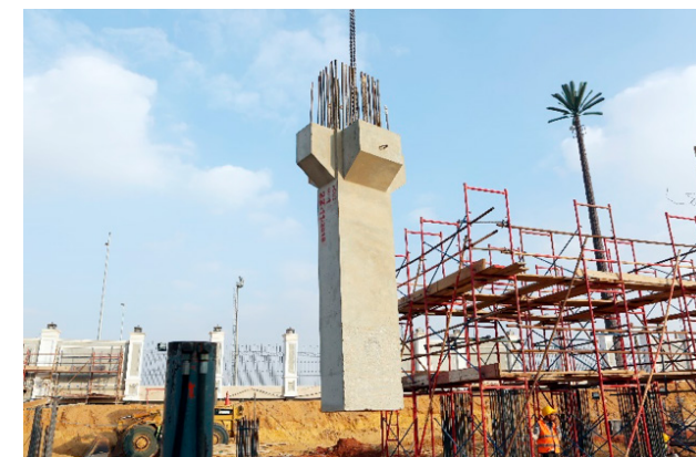
Figure 2.2 Sample of precast Column (by the Author)
