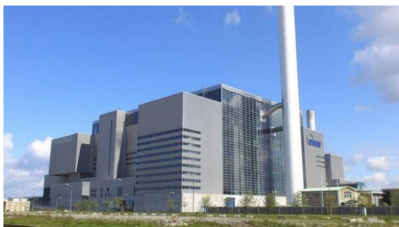
Figure 22. SYSAV in Malmö, Sweden (SYSAV's waste to energy plan, N.d.)
