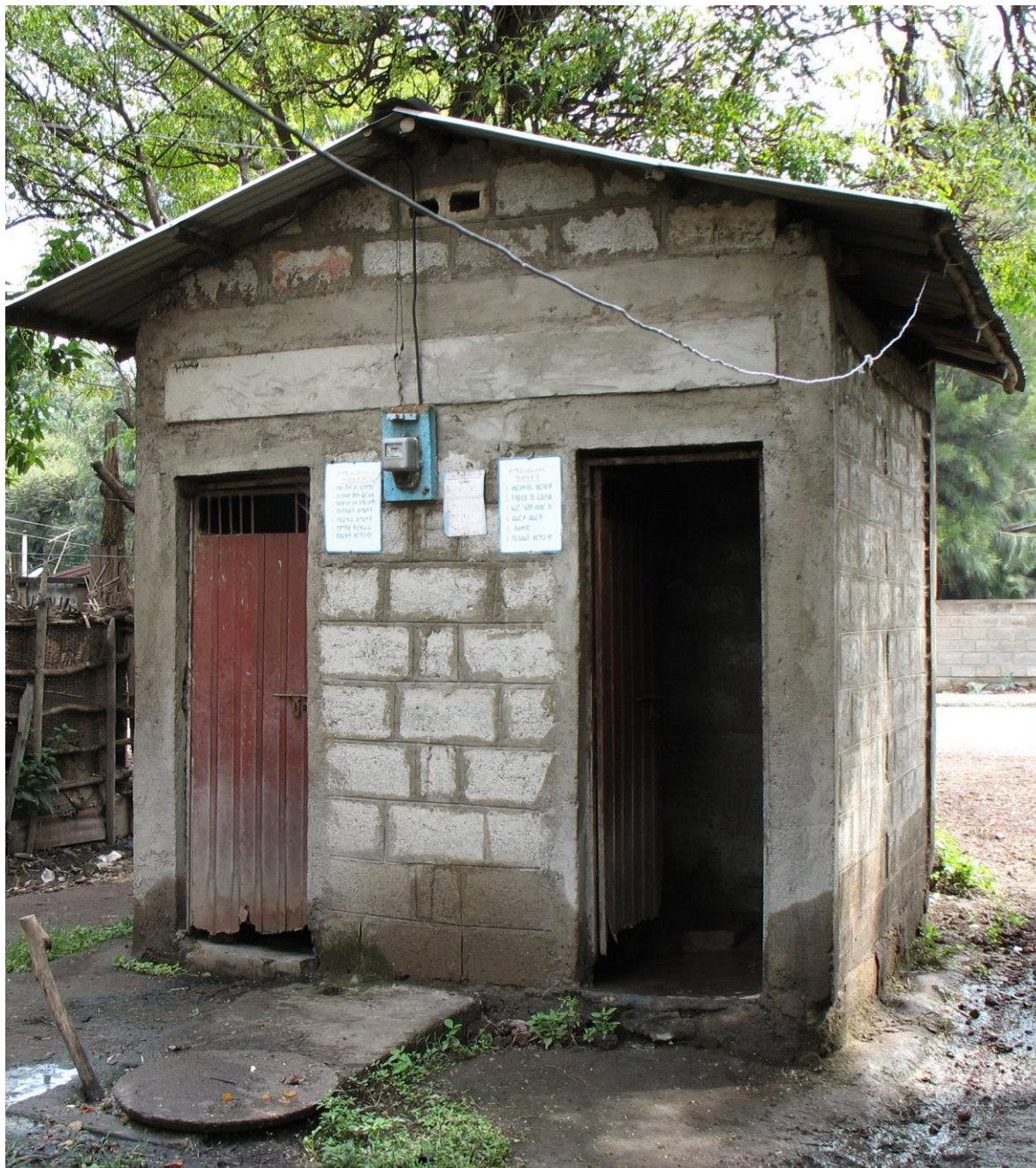
Picture 6: Women & Children Development Organization urban biogas toilet in Awassa, Ethiopia. The toilet has input hole for kitchen waste in the foreground.
