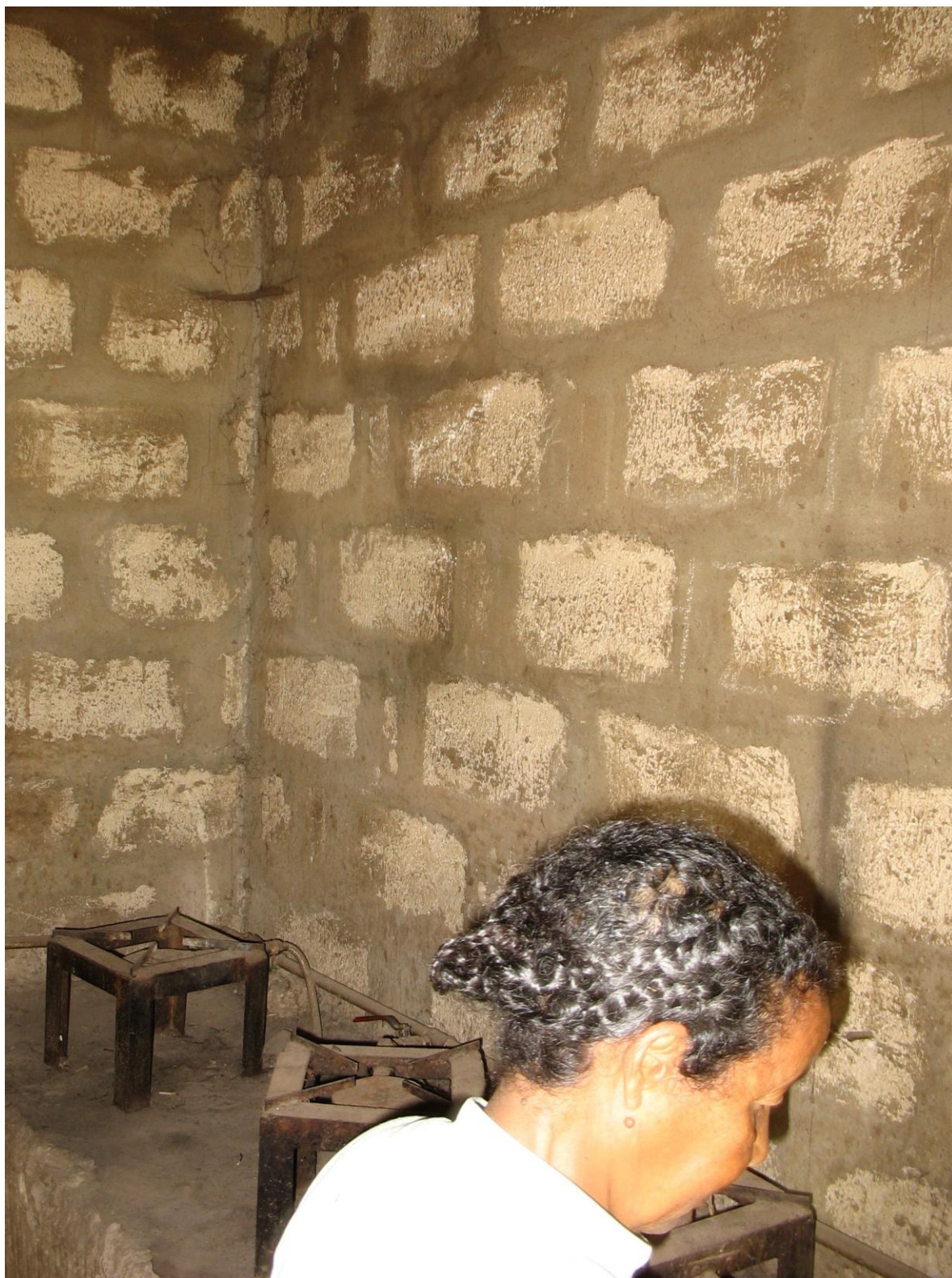
Picture 7: Woman cooking with biogas stoves in Awassa, Ethiopia. Burning biogas creates virtually no particulate matter, thus the kitchen walls and ceiling were clean of soot.
