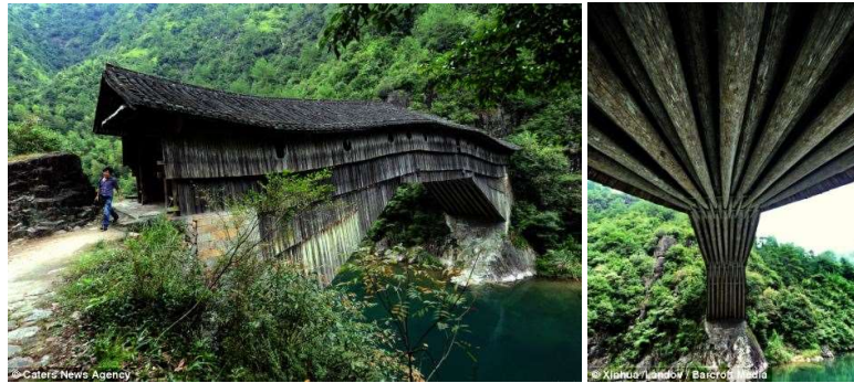
Figure 3. The Xianju Bridge in China (Wikimedia Commons, 2018)
