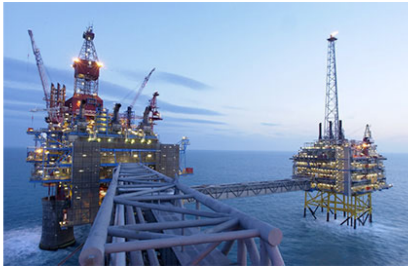
FIGURE 2. A platform for injecting CO 2 into safe, geological storage: Sleipner, Norway. Courtesy of Statoil. (ccs association 2012)
