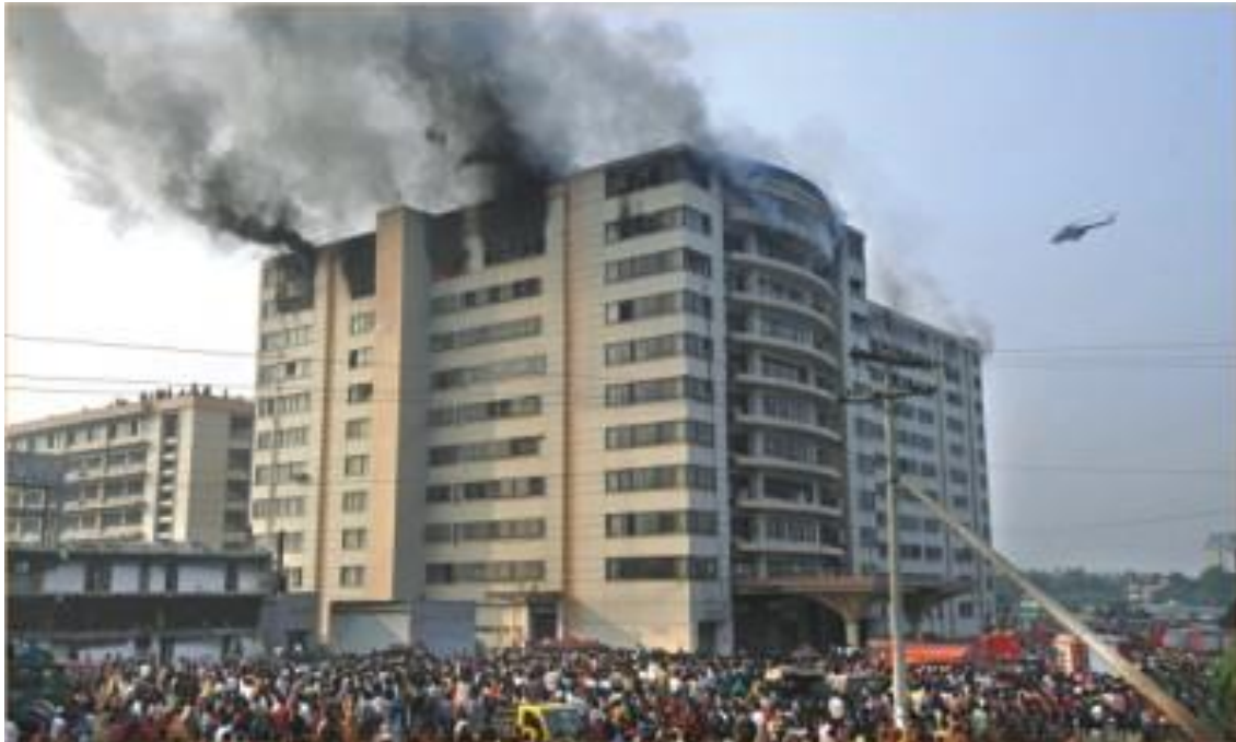
Figure 8: Ha-meem factory condition during the blaze (The Daily Star, 2010).
