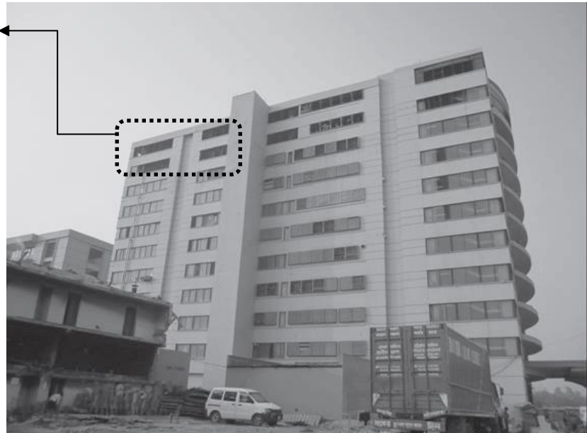
Figure 9: Factory view from outside (Sugahara, et al., 2011).
