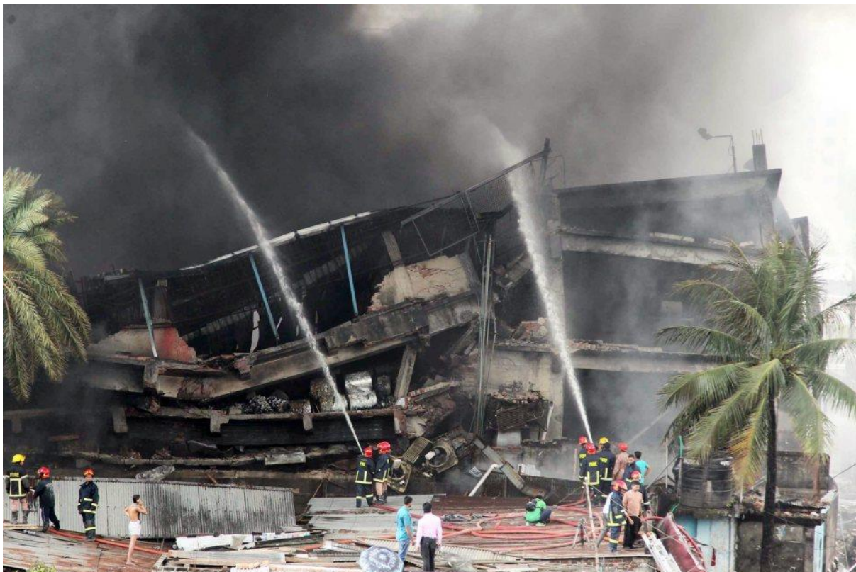
Figure 10: Distraction situation of Tampaco Foils Ltd. after the fire occurrence (The Sun, 2016).
