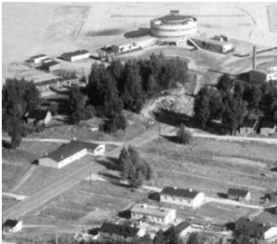
FIGURE 5. Courtyard area in 1951 (Freese & Schulman 2016).
