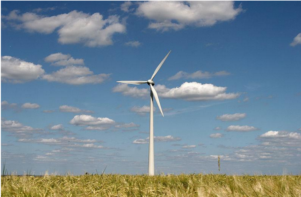
Figure 4. Wind turbine (W.Christian, 2006).
