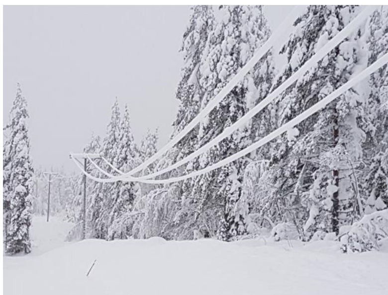
Figure 1. Enormous amount of wet snow stuck on trees and powerlines. Photo: Loiste Oy.
