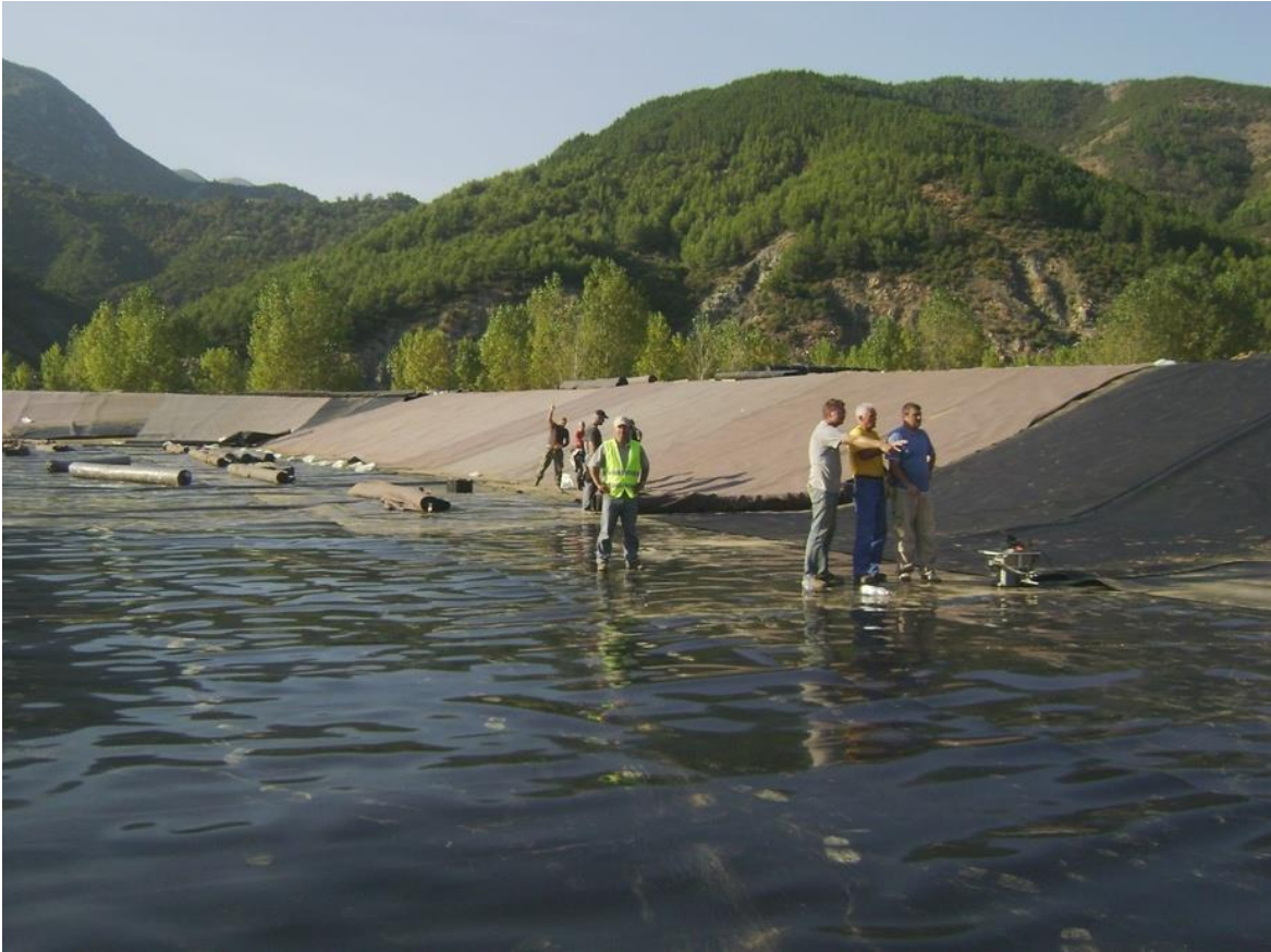
Figure 8. The process of geo-membrane and geo-textile placement (Mirdita Municipality, 2010).
