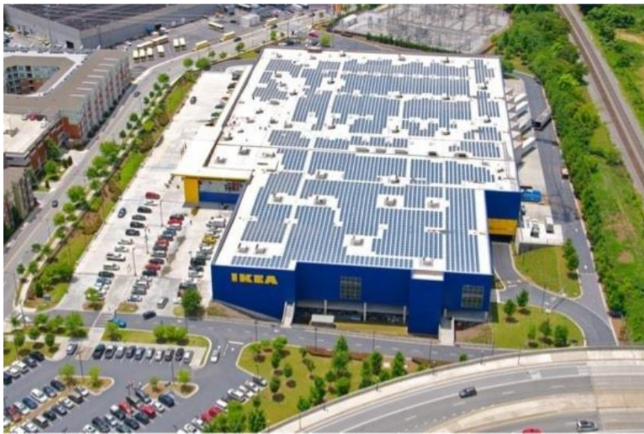
Figure 16. Solar panels on the roof of IKEA's shop in Boston, USA (Greenguruguides, 2014)
