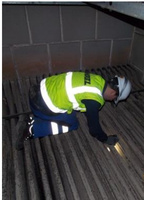
Figure 15. Visual inspection of tubes. (Andritz Oy's archives).
