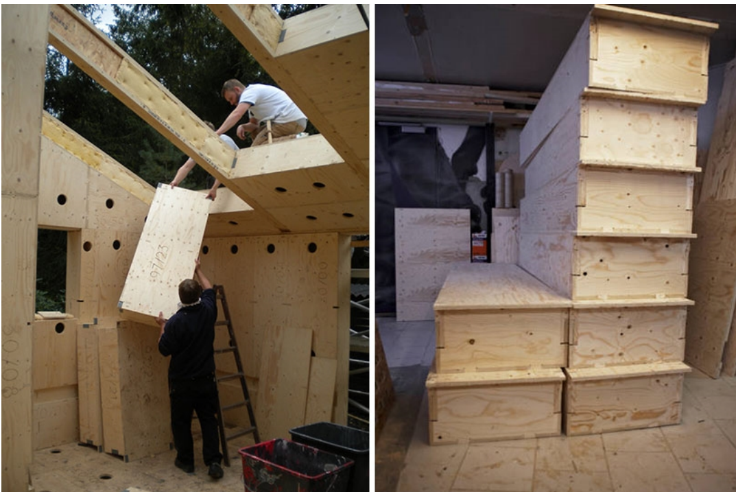
Figure 47. Modular segments and building process (Eentileen, 2012)
