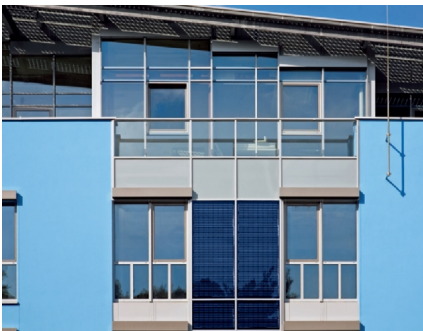
Figure 95. Solar modules (Schüco, 2017)
