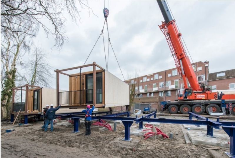
Figure 31. Placement of the module (Finch Buildings, 2017)
