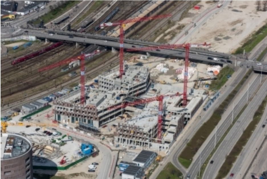
Figure 57. Progress building (A.Enggaard, 2015)
