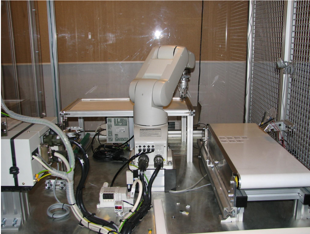
Figure 46: The new worktop installed.
